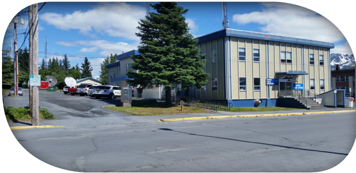
Figure 15 - City of Seward Police Station
