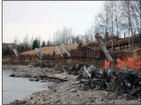
Image 1. Photo of the Kenai River boardwalk at Soldotna Creek Park. Photo courtesy City of Soldotna, 2009. Stairways are raised during the winter months to prevent damage due to flooding and ice flows.
