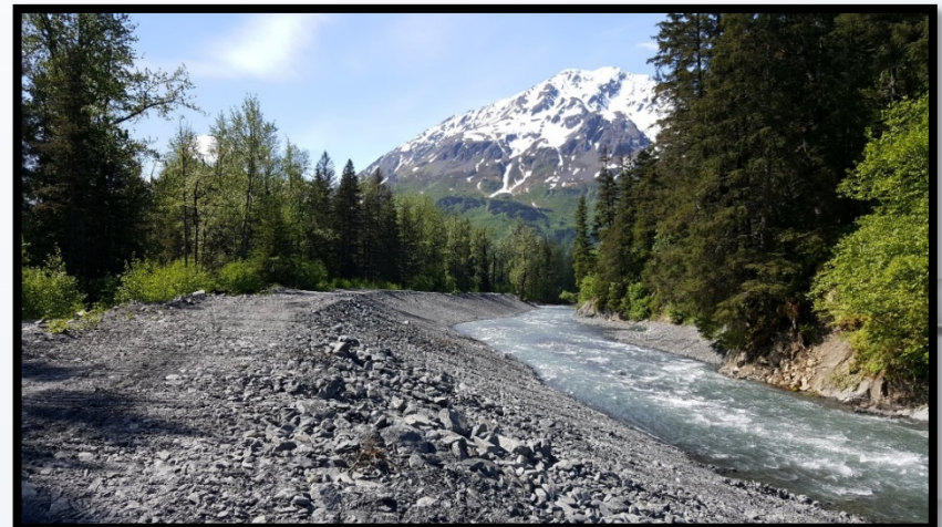
Box Canyon Creek Water Diversion Structure
