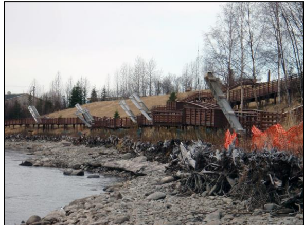
Image 1. Photo of the Kenai River boardwalk at Soldotna Creek Park. Photo courtesy City of Soldotna, 2009. Stairways are raised during the winter months to prevent damage due to flooding and ice flows.
