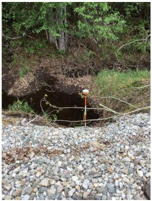
Photo 1. MP 30.44 culvert inlet area (buried)
