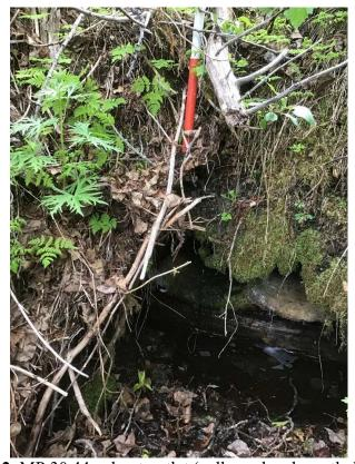
Photo 2. MP 30.44 culvert outlet (collapsed and mostly buried)
