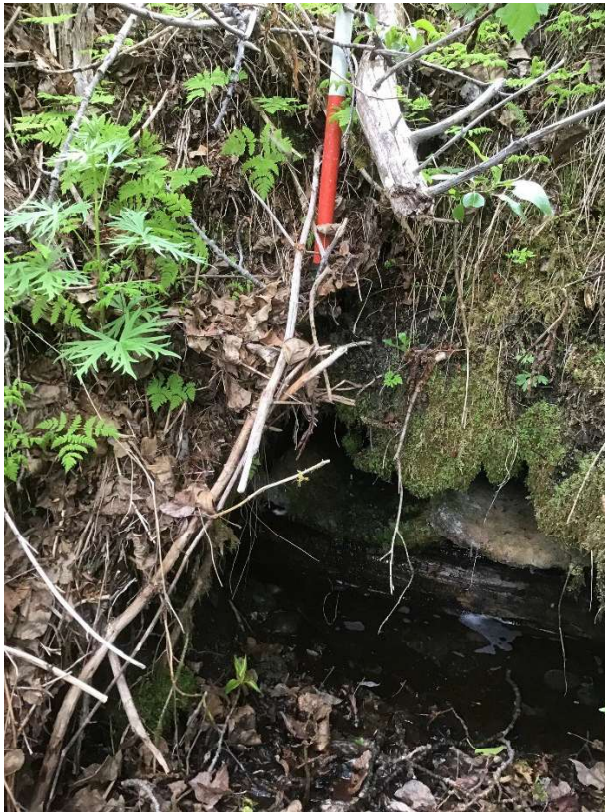
Photo 2. MP 30.44 culvert outlet (collapsed and mostly buried)
