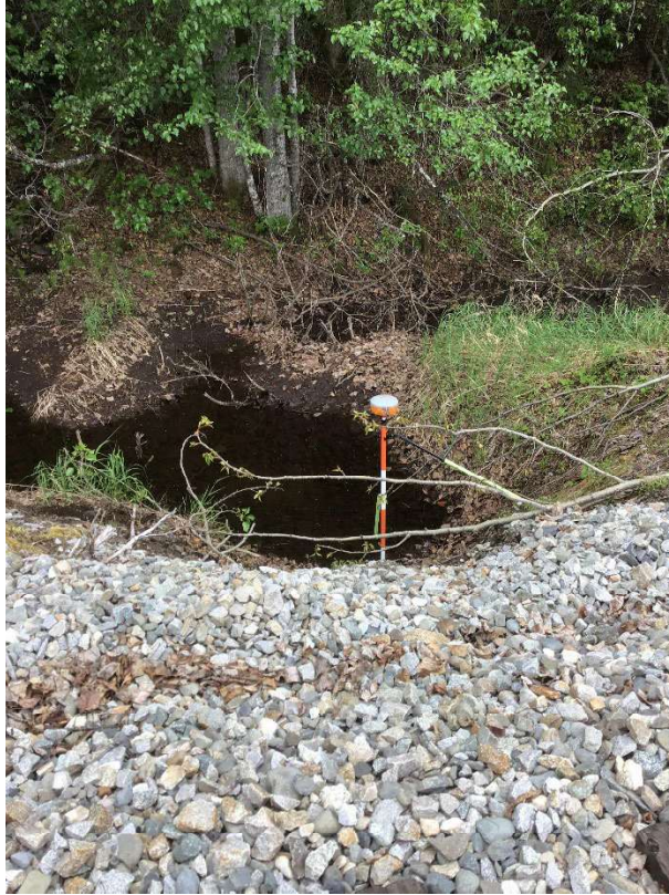
Photo 1. MP 30.44 culvert inlet area (buried)
