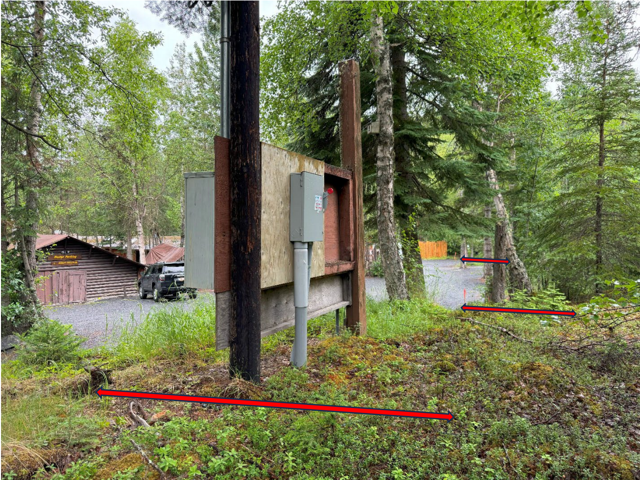
Annotated arrows from visible property edge stakes are approximate and illustrative only. Main utility pole and meter base has been in continuous operation since before the ROW was platted.
