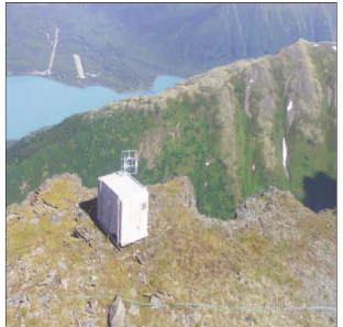
2 Aerial View of Kenai Peninsula Borough Building with cable along ground
