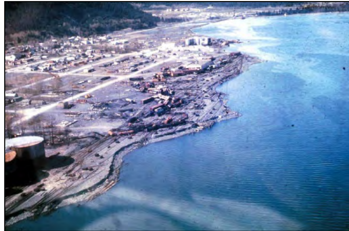
Tsunami damage to Seward Infrastructure after 1964 Earthquake (USGS)
