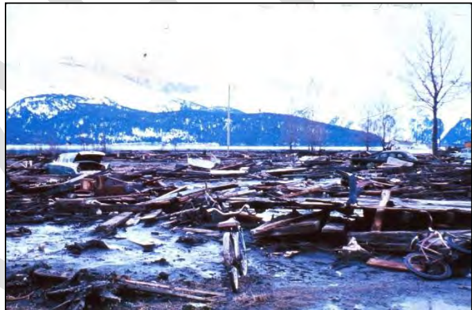
Tsunami damage in Seward after 1964 Great Alaska Earthquake (USGS)
