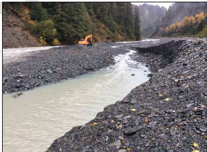
Flood mitigation efforts after severe flooding in Seward, October 2020
