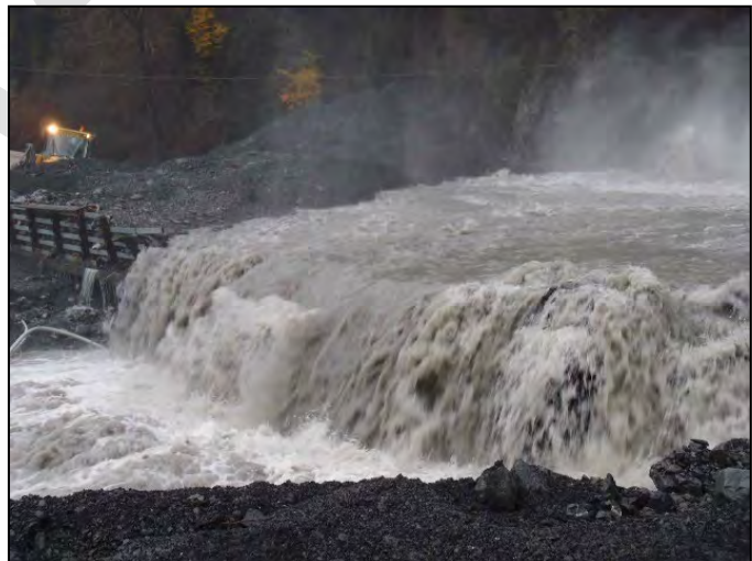
Flash flood event at the Lowell Creek Tunnel outflow in Seward (City of Seward)
