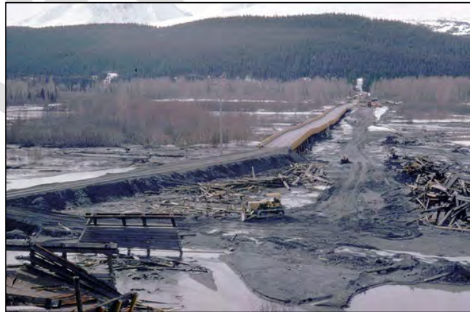
Damage to the Seward Highway from the 1964 earthquake. (UA Archives)
