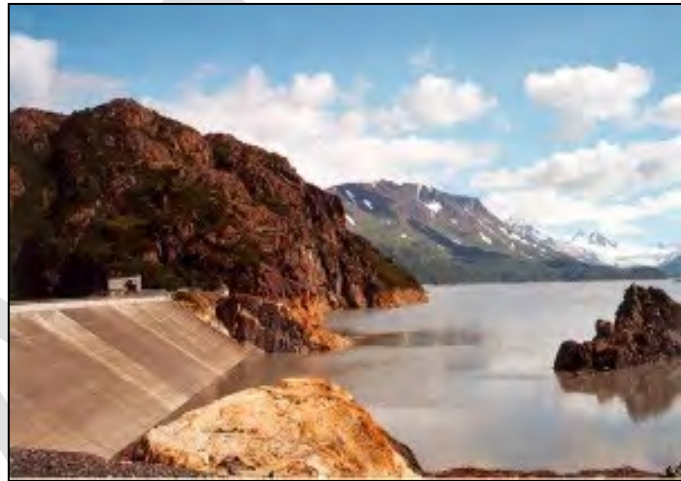
Bradley Lake spillway dam and hydroelectric plant near Kachemak Bay in the KPB. (HEA)
