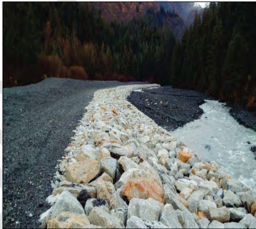
SBCFSA Salmon Creek Revetment Project
