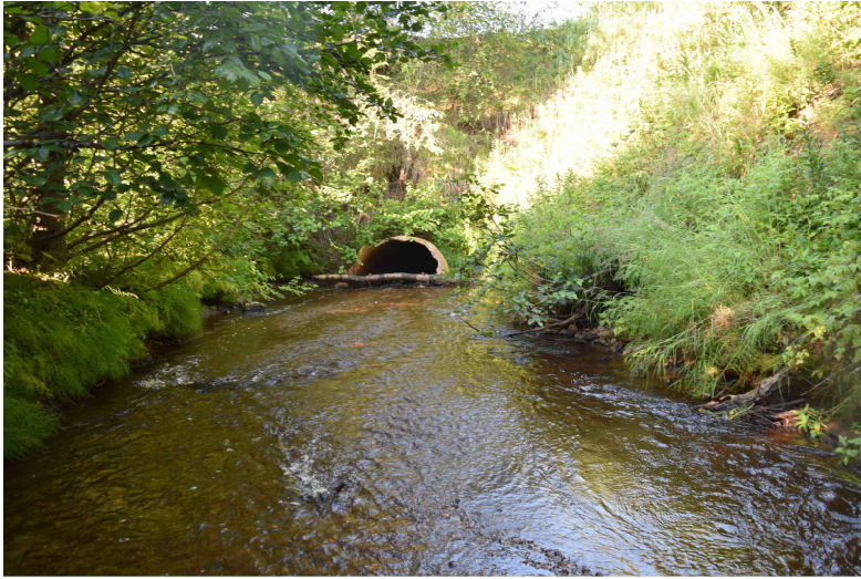
EXISTING CULVERT INLET
