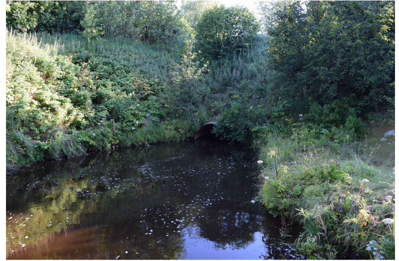
EXISTING CULVERT OUTLET
