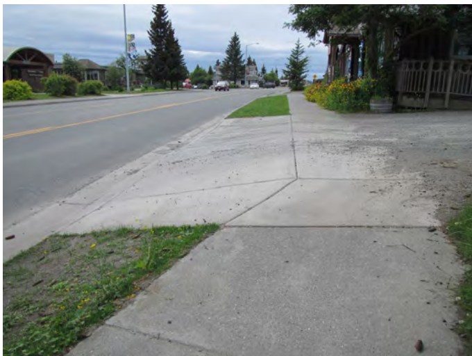
Figure 19: Driveway Entrance with Level Cross Slope
