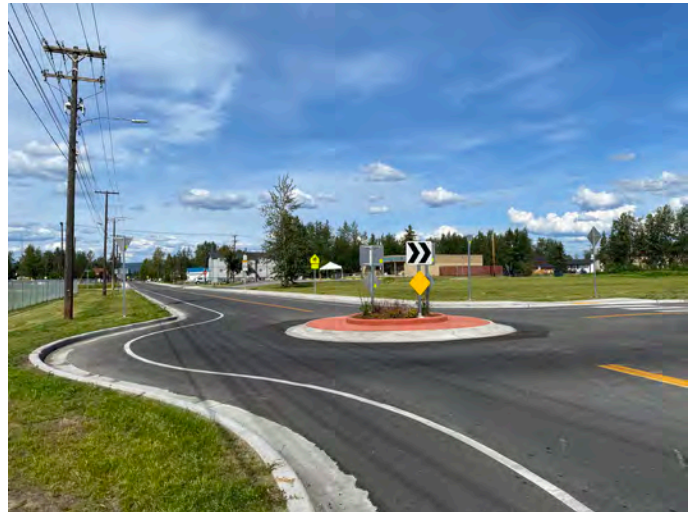
Figure 25: Traffic Circle on Gillam Way in Fairbanks
