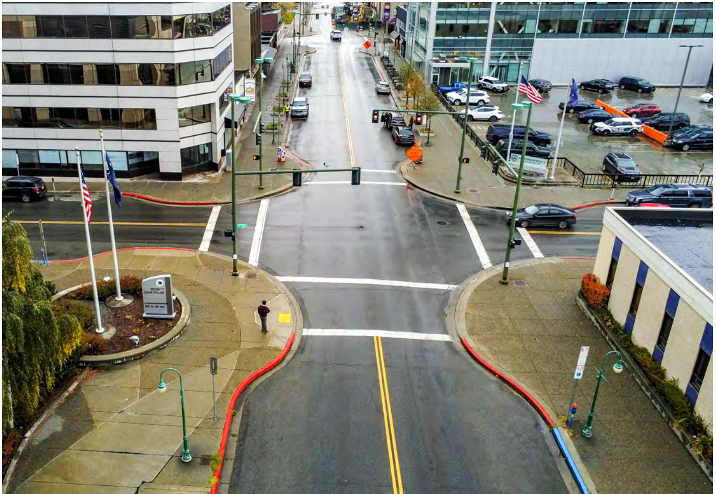
Figure 24: Curb Bulb-outs in Downtown Anchorage, Alaska
