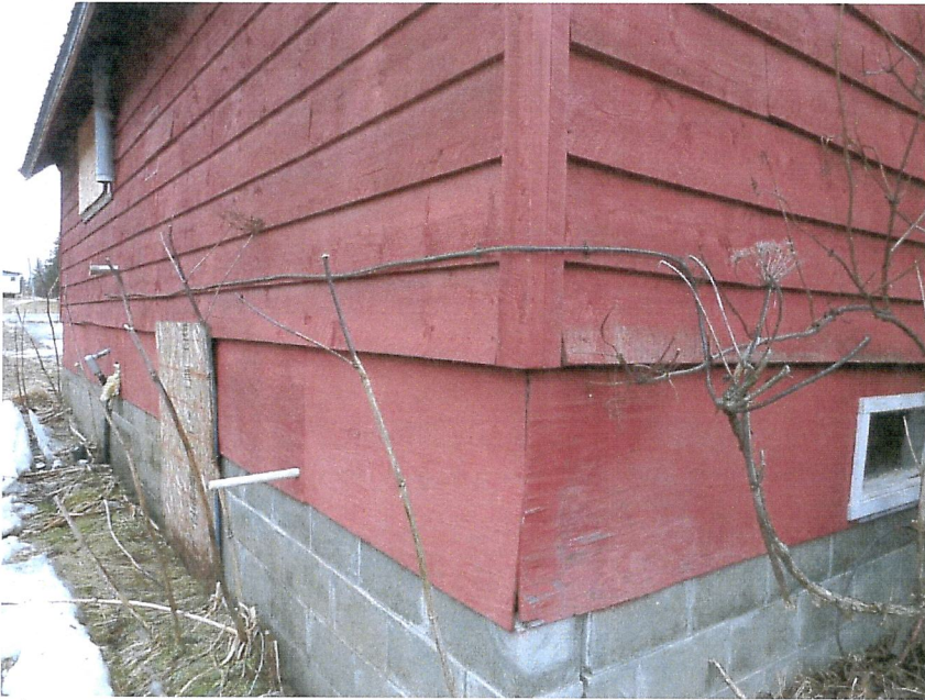
Photo 8: One of the Two Fuel Lines
