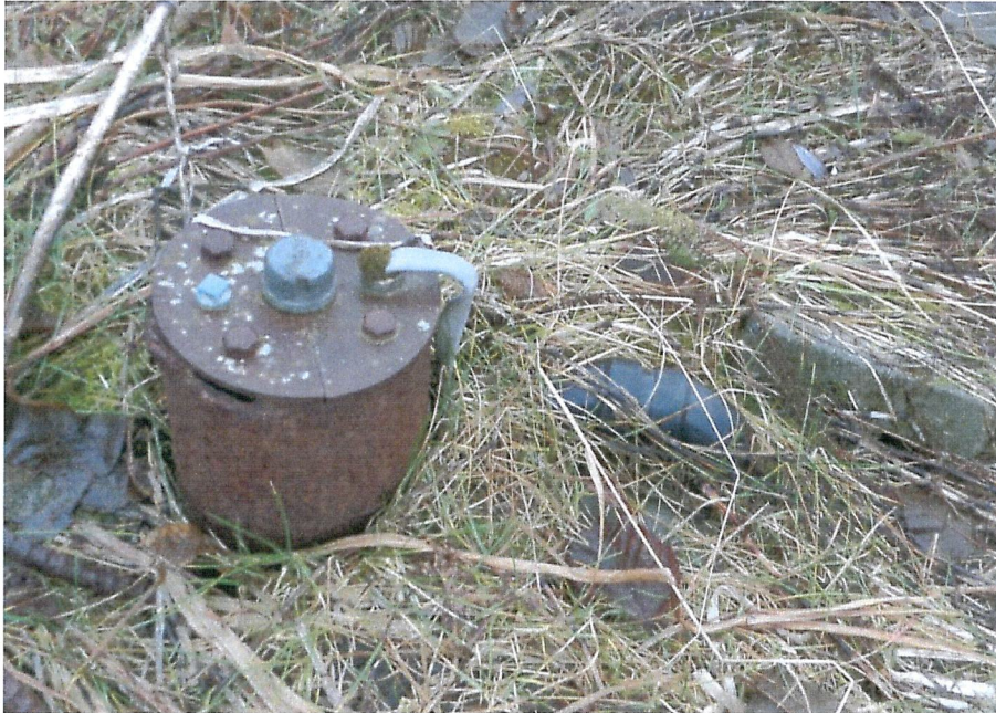
Photo 1: Wellhead (in need of improvements if used as a potable source)
