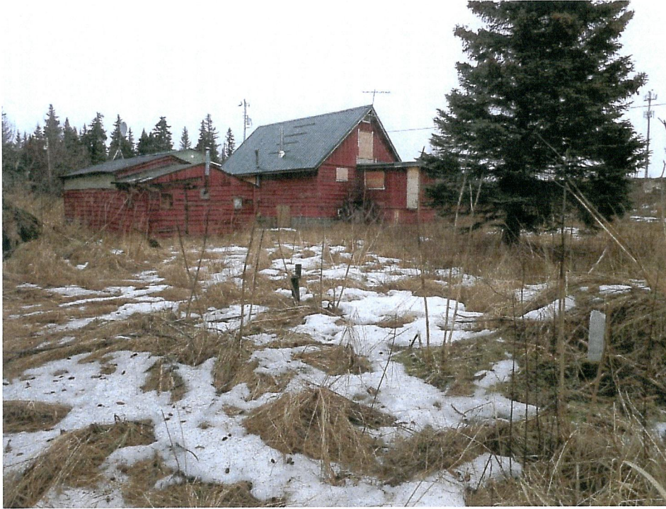
Photo 3: Septic Tank Risers ( center of photo ) and Broken Possible SAS Riser ( right side )
