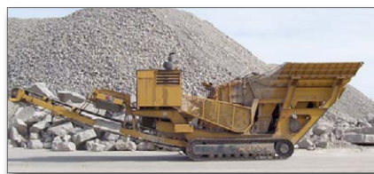
Figure 6. Crushed concrete stockpile and crusher
