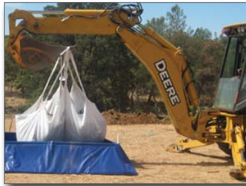
Figure 12. Extracting the concrete solids or gelled washwater
