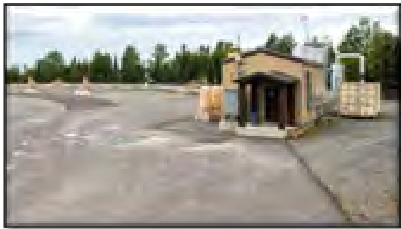
Gas Facility in Kenai
