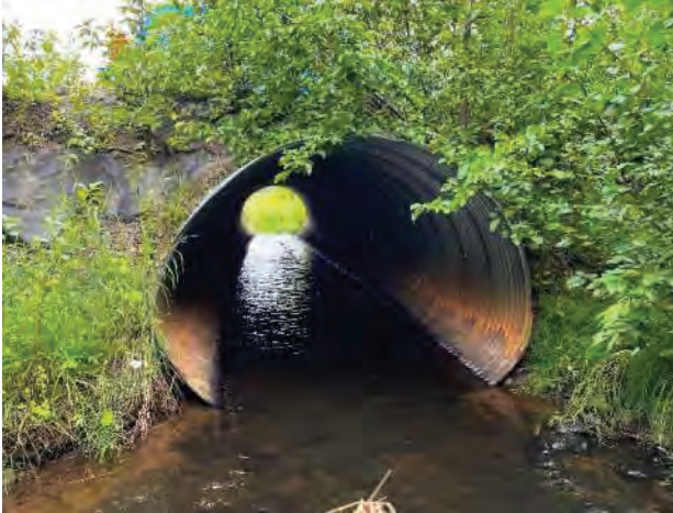
North Culvert Outlet (facing upstream)
