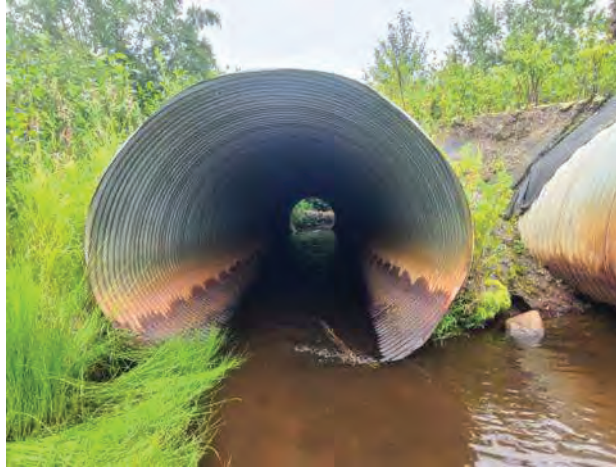
South Culvert Outlet (facing upstream)
