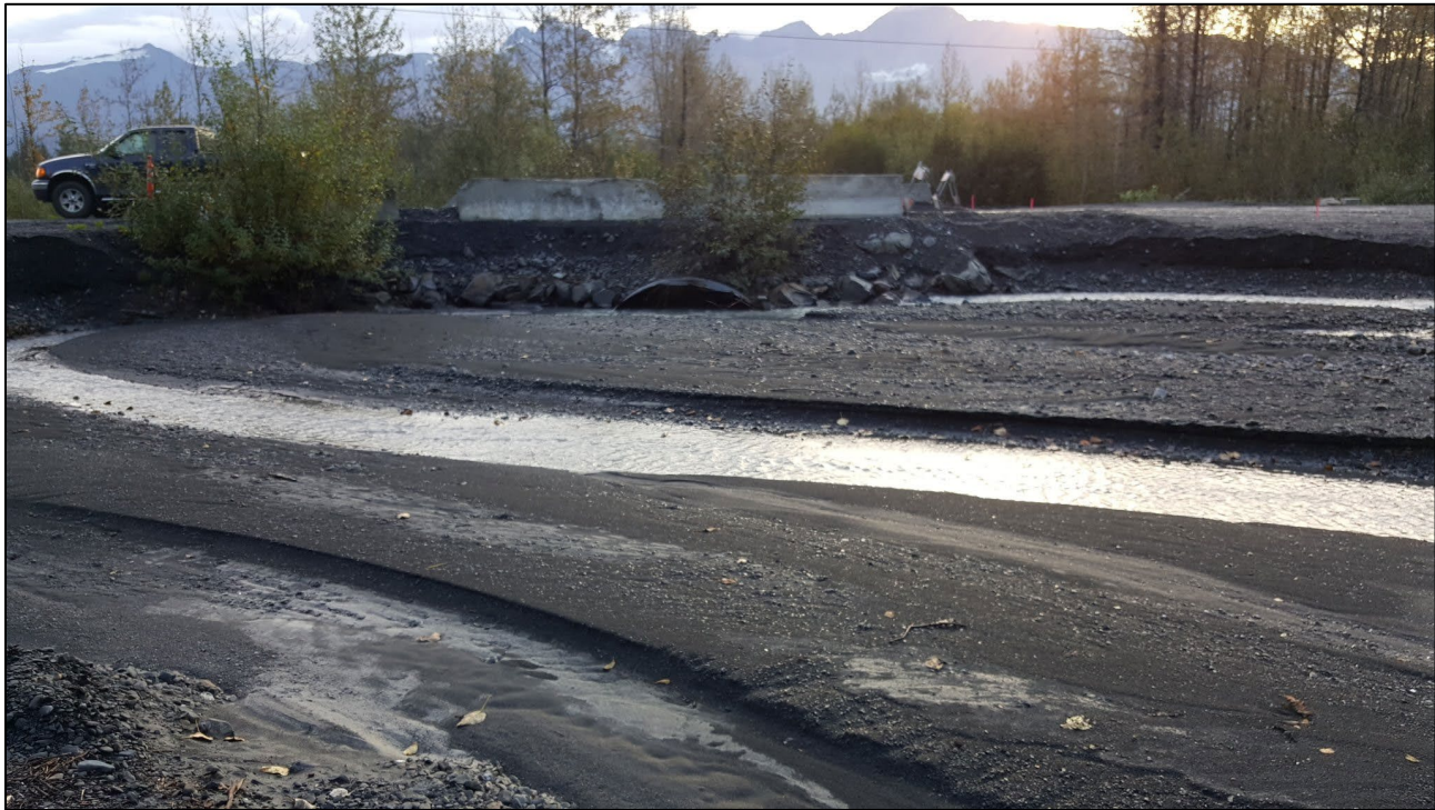
Figure 5. Main 12' culvert under Dieckgraeff Road.
