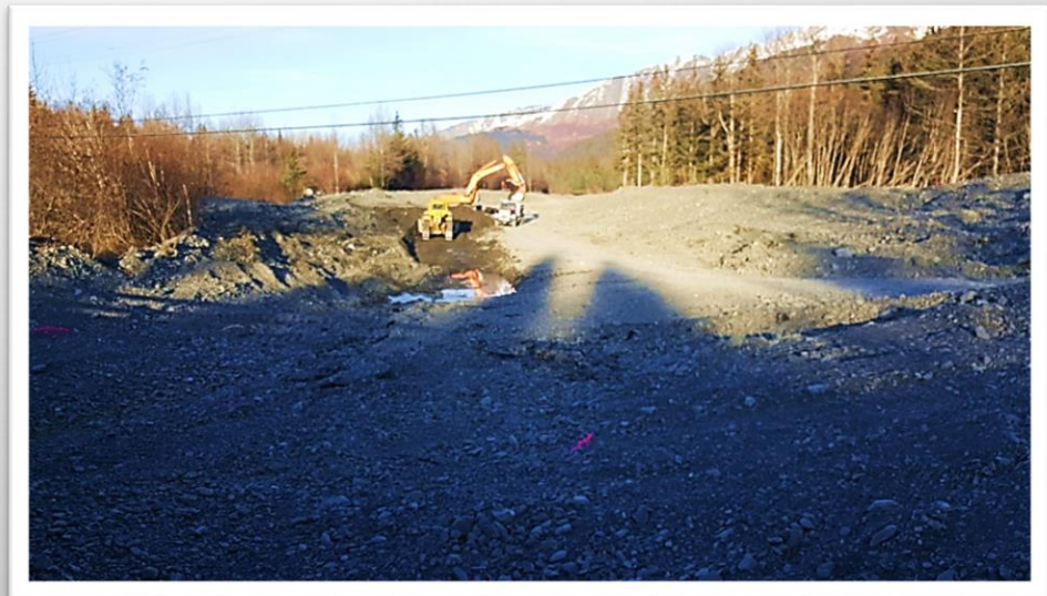
Sawmill Creek maintenance project, following 2020 flood event.
