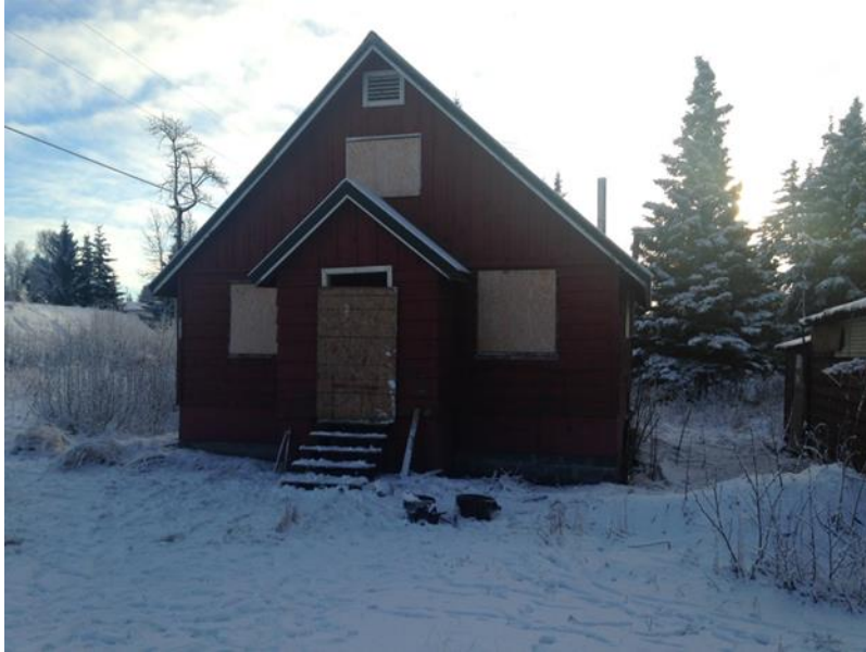
Existing Residential Structure.
