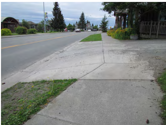
Figure 19: Driveway Entrance with Level Cross Slope
