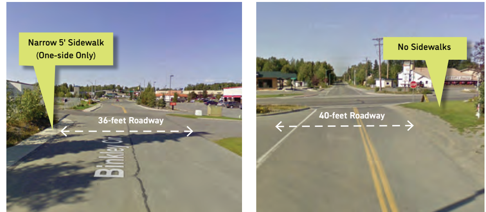
Fig. 77: Partially Improved Streets- Binkley Circle & Birch Street
