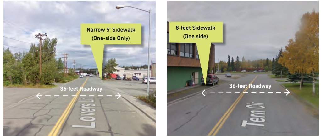
Fig. 75: Partially Improved Streets (Lover's Lane & Tern Circle)
