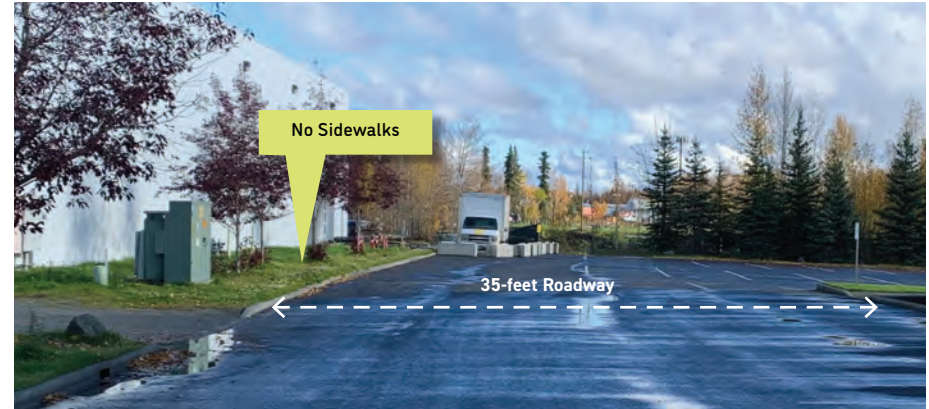
Fig. 71: Existing Driveway at Aspen Hotel (Looking Northeast)
