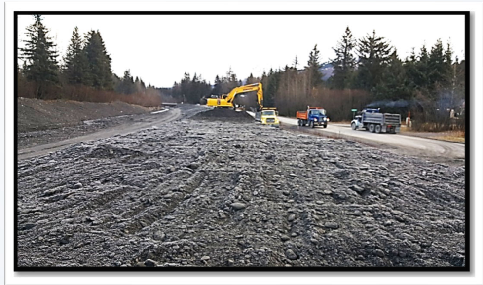
Kwechak Creek sediment management & maintenance project.
