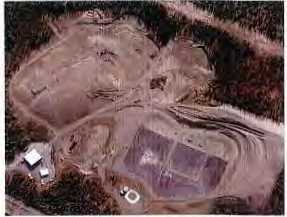
CPL Lined Cell #1 Construction (2005)
