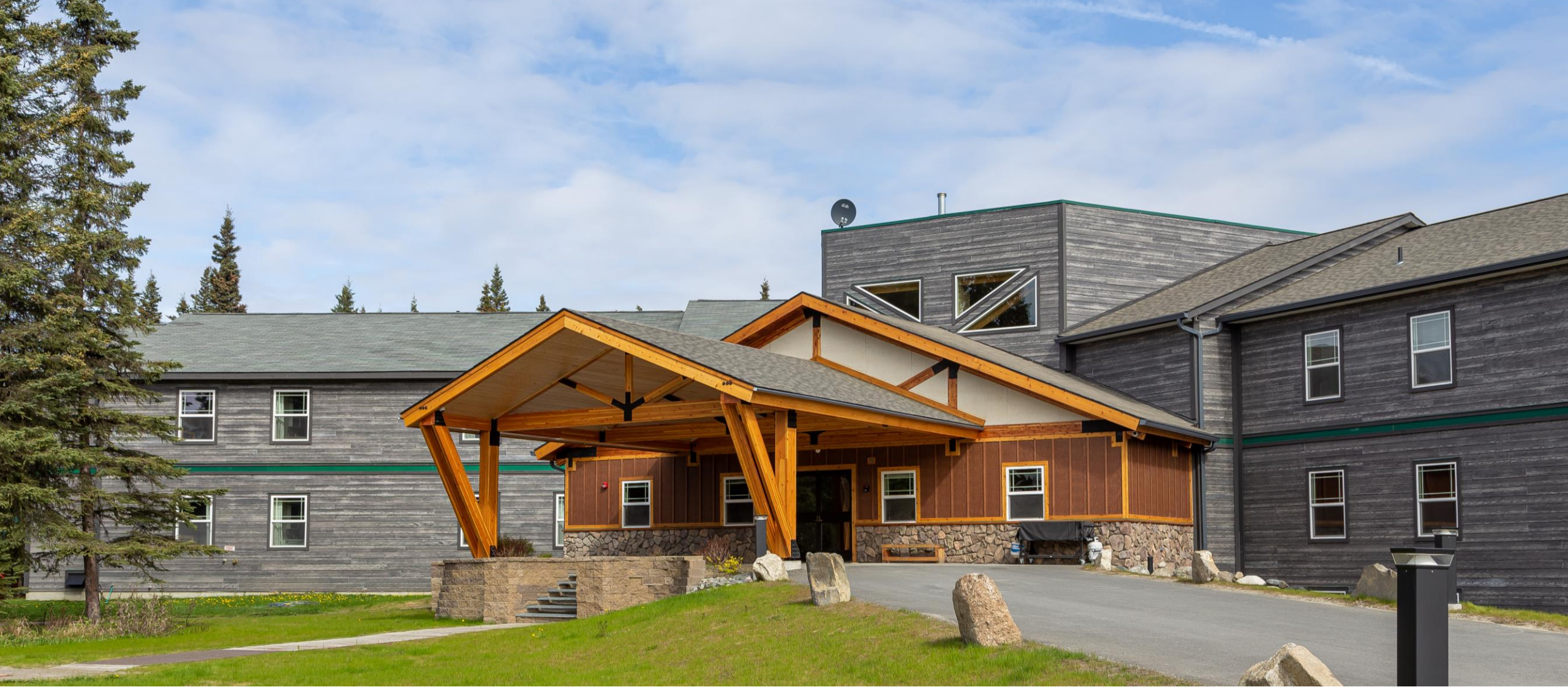
Peninsula Conference Center and 64-bed dormitory completed in 2018
