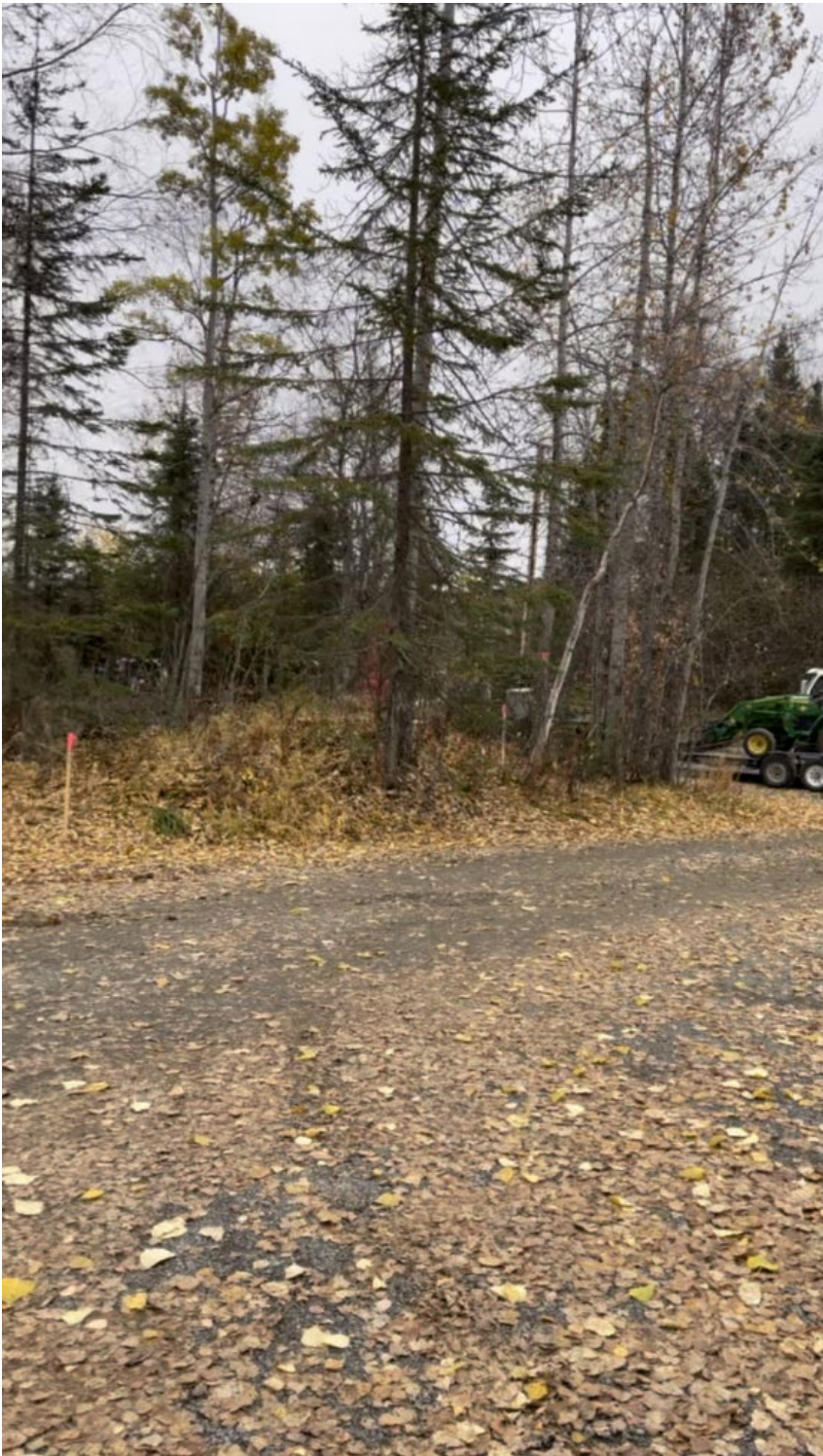
Attachment # 6 Survey stakes of Lot 10 before construction began.
