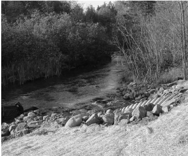
Erosion mat and rock are two effective ways to control erosion.
