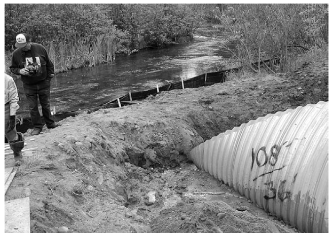
Control erosion during and after construction.
