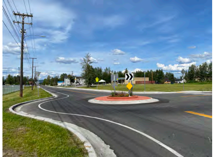
Figure 25: Traffic Circle on Gillam Way in Fairbanks
