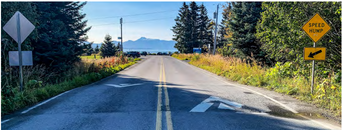
Figure 23: Speed Hump on Beluga PI
