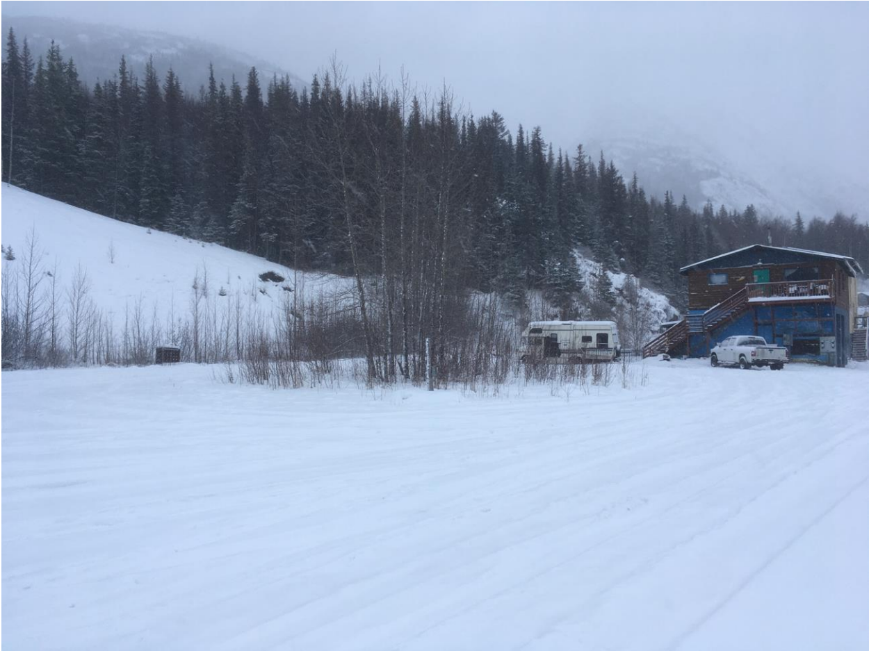
Photograph #1: View of failed slope from the Sterling Highway. Affected structure on the right.
