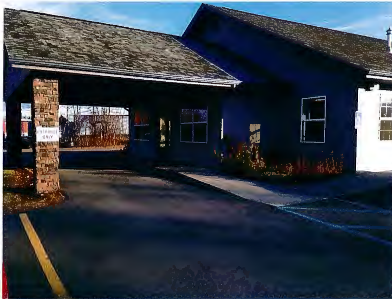
Photo 1: Entry showing handicap ramps and HC parking sign
