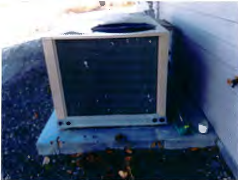
Photo 5: Gas fired, ground mounted, package HVAC unit.
