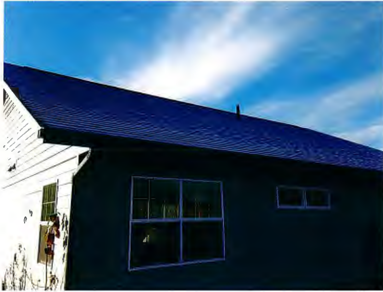
Photo 4: Frost on roof showing ventilation and insulation quality.
