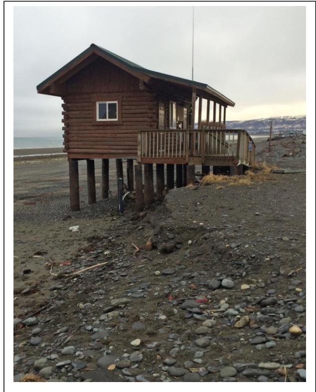
Above: In the fall of 2015, the City had this camp host building removed from the west side of the Homer Spit. Previous attempts to reduce the impact of coastal storms were not successful.
