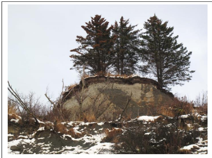
Looking up from the beach, chunks of land slough downward toward the shoreline.
