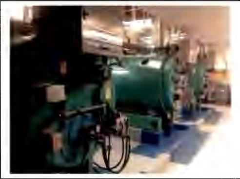
**Fig.2:** CB boilers fitted with door conversions and Riello burners.
