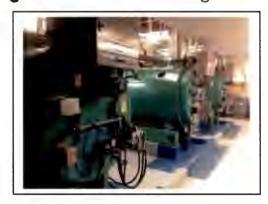
Fig.2: CB boilers fitted with door conversions and Riello burners.
