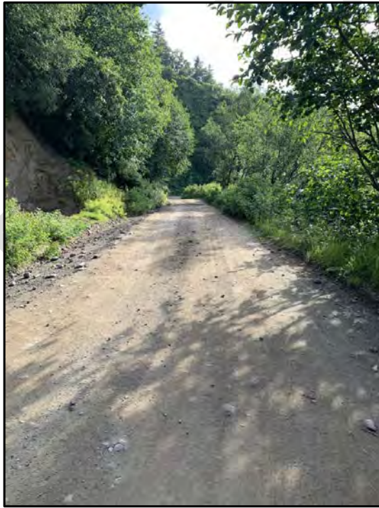
Figure 2.14. Narrow unsurfaced road that may make fire response difficult.
