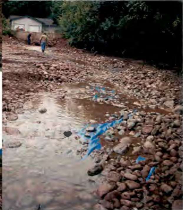
Digging of outlet stream channel, laying of impermeable fabric and initial stream shaping in July 2006.
