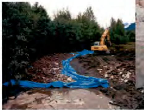
Digging of outlet stream channel, laying of impermeable fabric and initial stream shaping in July 2006.
