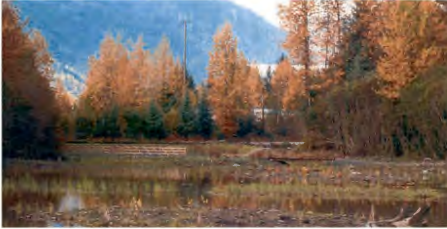
The finished bridge and boardwalk cross the wetland to an island with a bench for viewing.
