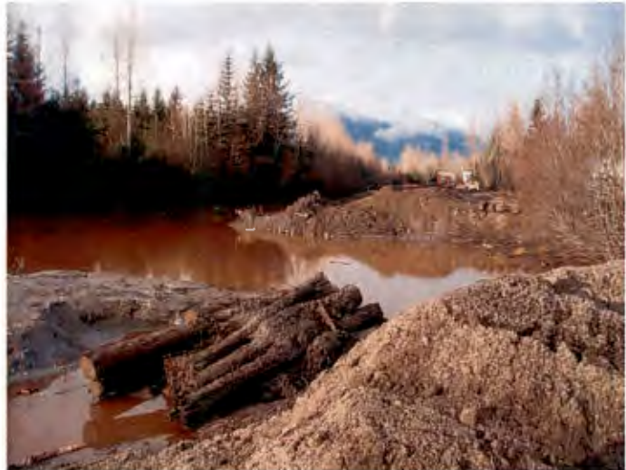
Early stages of filling in November, 2005. Logs are used to support machinery as the fill the fingers.
