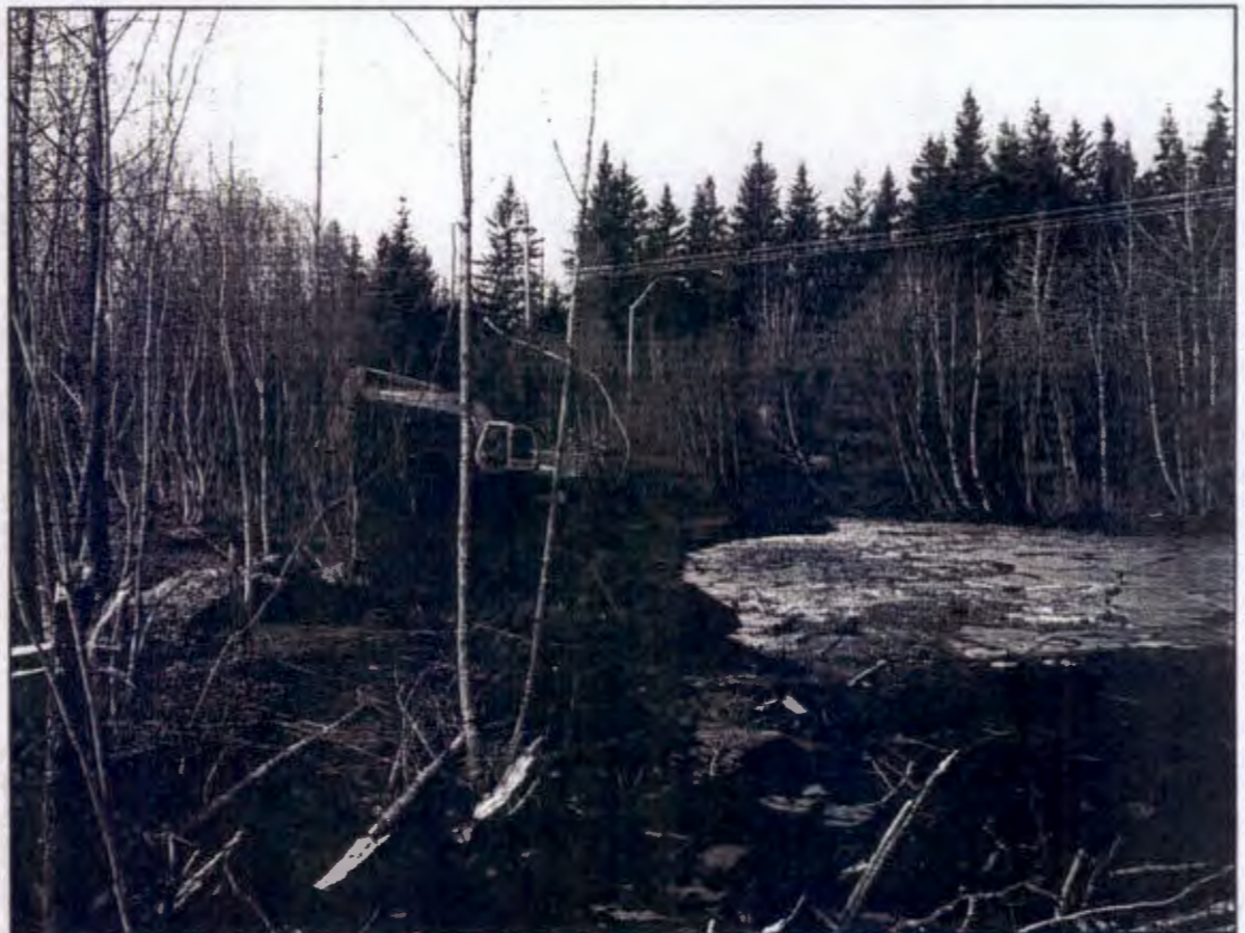
Emergent wetlands are created along the perimeter of a deep water pool for juvenile coho salmon habitat.
