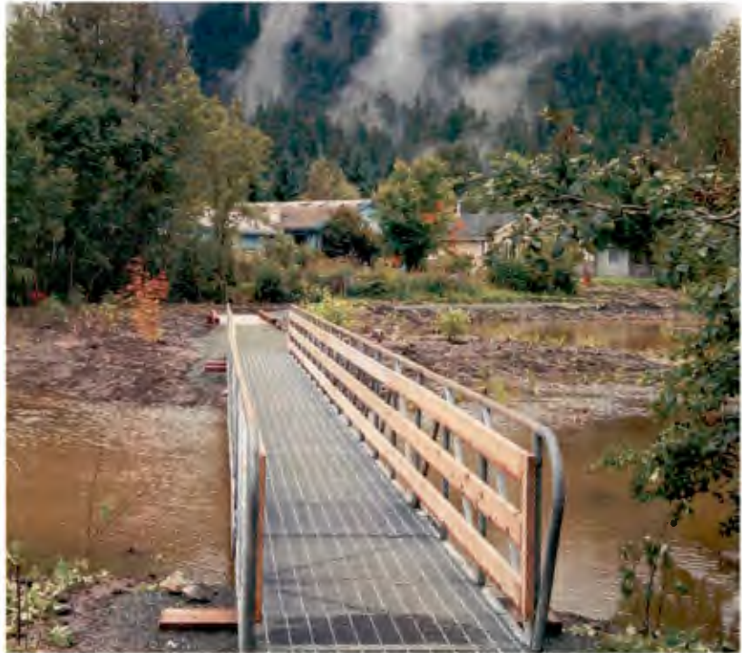
Right: The steel gangway donated by CBJ Ports and Harbors extends from the northwest end of the trail to the east side. Trail Mix built new cedar rails for safety.
