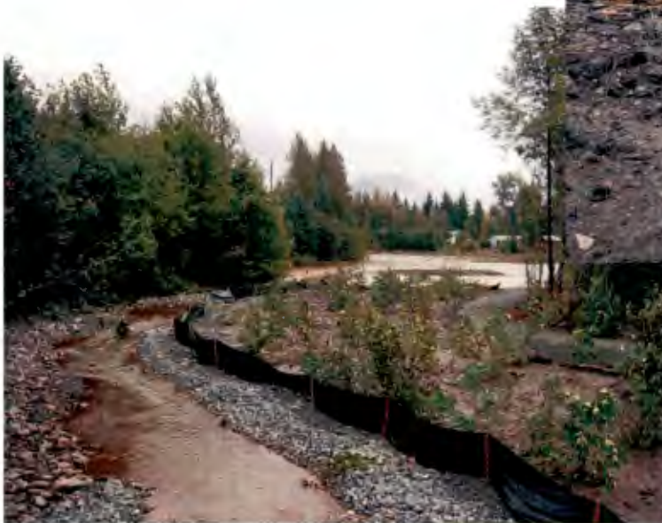
Left: Alders transplanted along stream channel.
