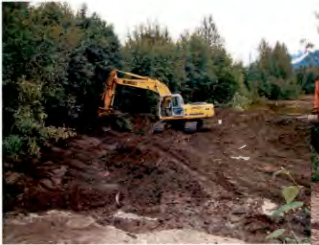
Digging of outlet stream channel, laying of impermeable fabric and initial stream shaping in July 2006.
