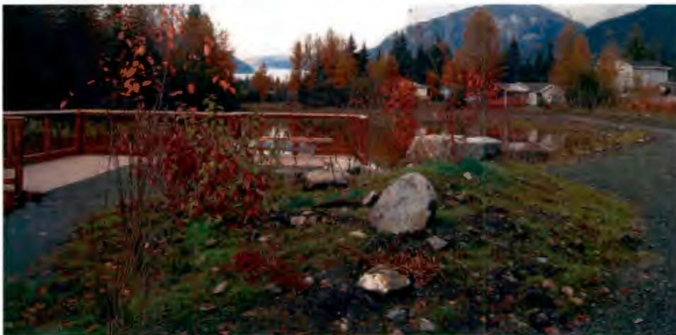
Below: The finished observation deck and gathering area.
