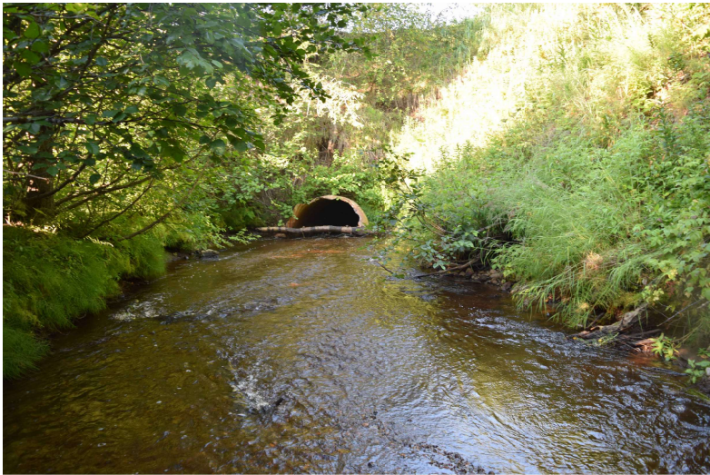
EXISTING CULVERT INLET
