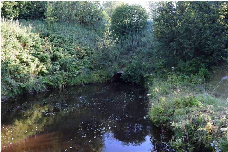
EXISTING CULVERT OUTLET
