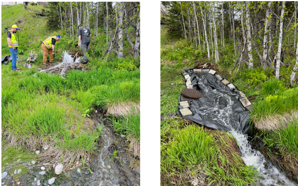
Figure 2. Site of collapsed pipe and associated manhole.
