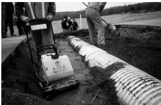
Adequate compaction is essential to culvert installation. Hand tamping is often best.
