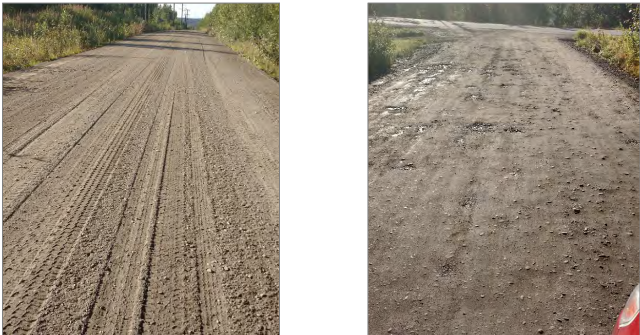
Figure 4 – Left: Gravel Road in Good Condition (Rating 8) / Right: Gravel Road in Poor Condition (Rating 4)
