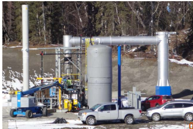
Figure 51. Installing Leachate Evaporation System, Central Peninsula Landfill
