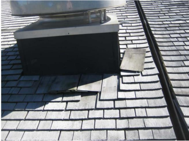
Shingles broken and sliding out of position.
