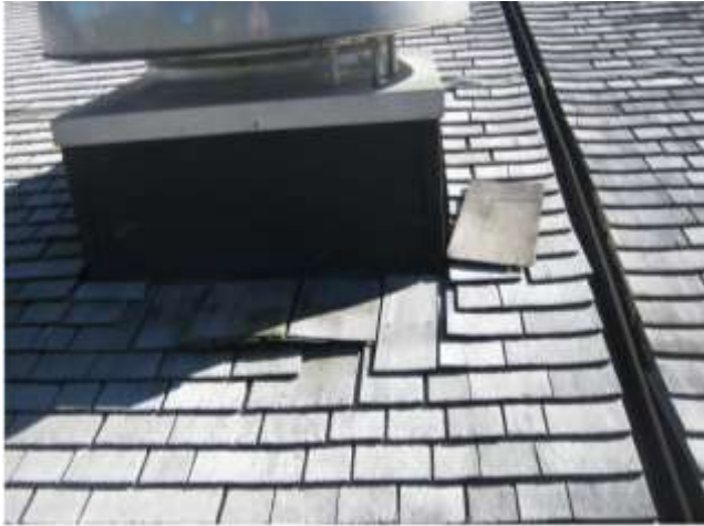
Shingles broken and sliding out of position.
