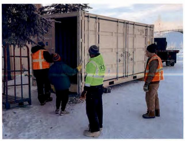
A shipping container provides the basic structure for the kitchen-bathroom module. (Courtesy of Cold Climate Housing Research Center)
