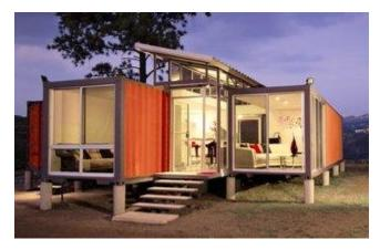
Made of scraps taken from the containers' sides, the roof creates a sense of openness from the inside and ushers in sunlight. Its slanted design creates a wind tower effect, providing natural ventilation that negates the need for air conditioning.
