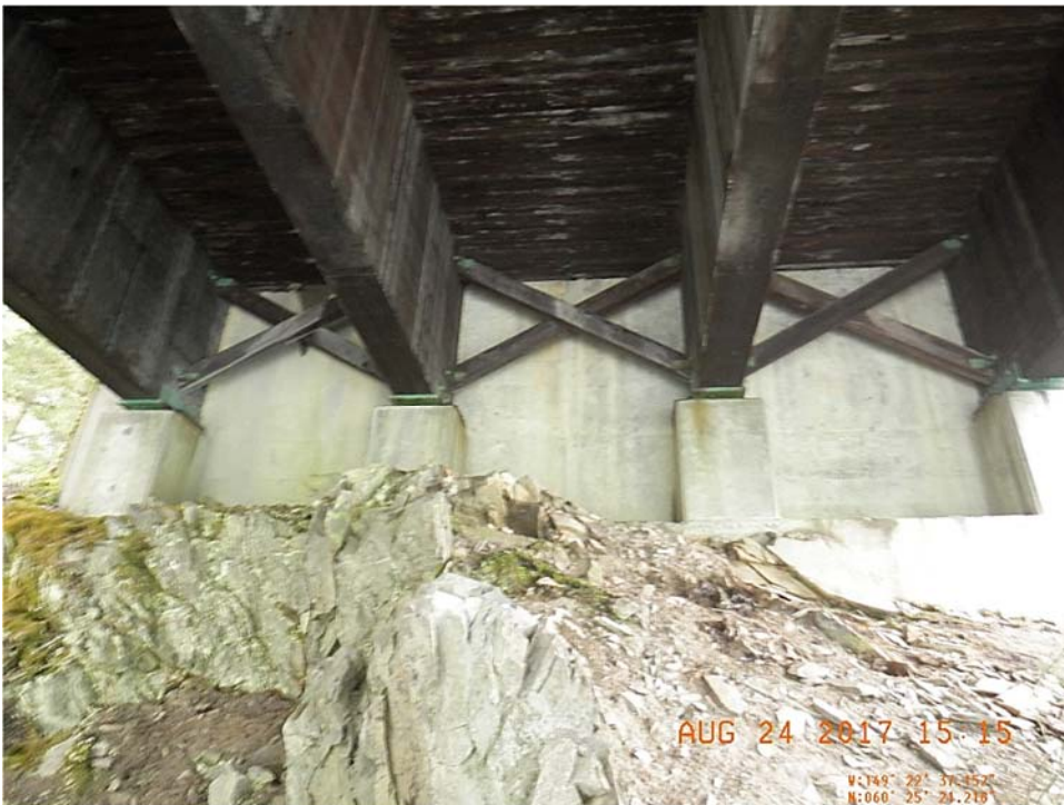
Existing abutments cast onto bedrock
