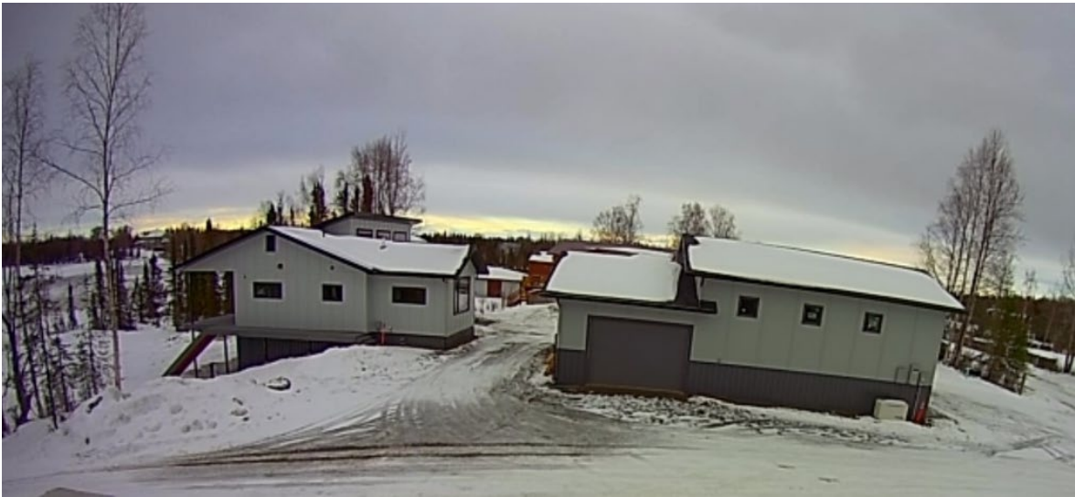
Attachment #12 Gutter draining into GL Hollier creating icy road conditions.
