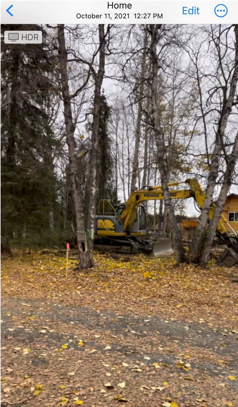
Attachment #5, Survey stakes on Lot 10 before construction began.
