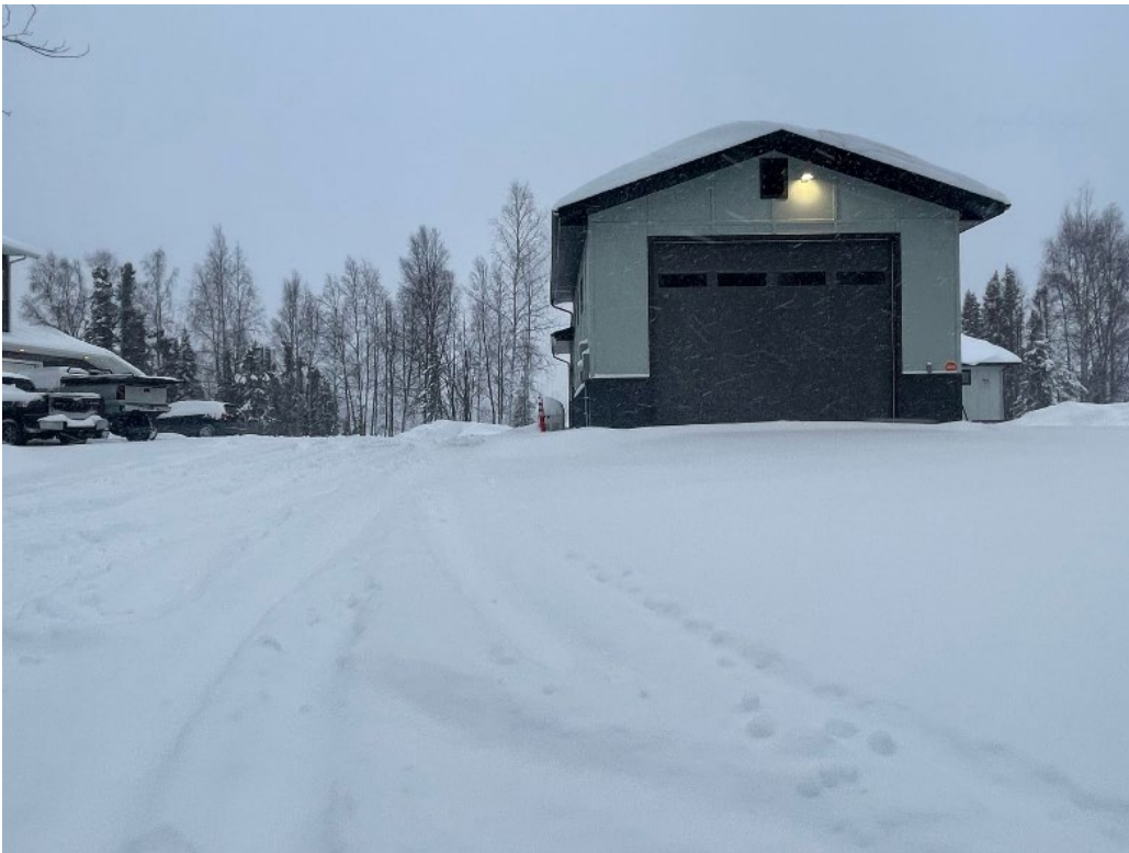
Attachment #2, Generator beside shop in setback.
