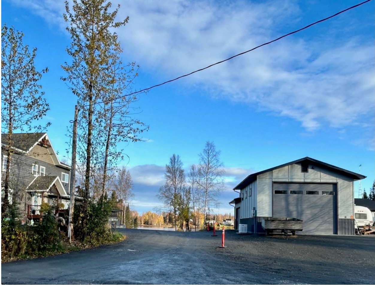
Figure 5. View from south side of Ross Drive towards GL Hollier Street and our garage (right); cones indicate lot line.
