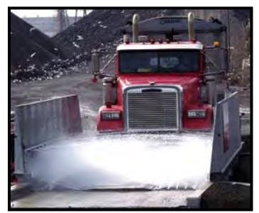
Figure 8-5: Wheel Washer with Sprayers (Photo from January-February issue of Erosion Control Magazine article "Controlling Fugitive Dust on Roadways" by Carol Brzozowski)
