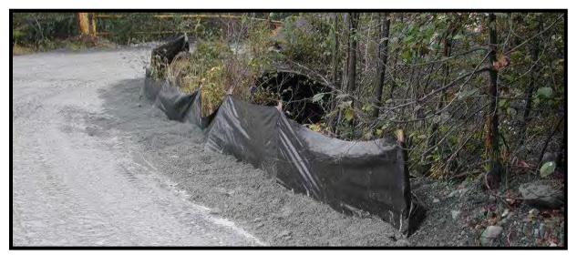
Figure 7-8: Silt Fence Example (Photo: City and Borough of Sitka)
