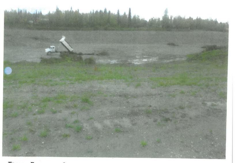
TRUCK DUMPING ORGANIC RECLAMATION MATERIAL INTO THE OPEN WATER AQUIFER IN SBC PIT SEPTEMBER 2014
