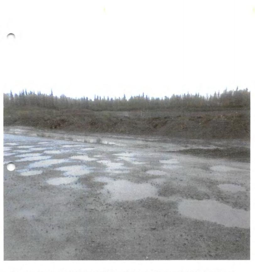
**CLOSER VIEW OF BOROUGH ROAD DAMAGE FROM SBC PIT ACTIVITY** SEPTEMBER 2014
