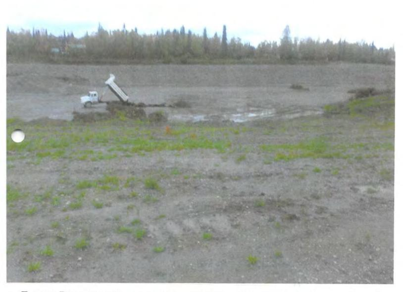
TRUCK DUMPING ORGANIC RECLAMATION MATERIAL INTO THE OPEN WATER AQUIFER IN SBC PIT SEPTEMBER 2014
