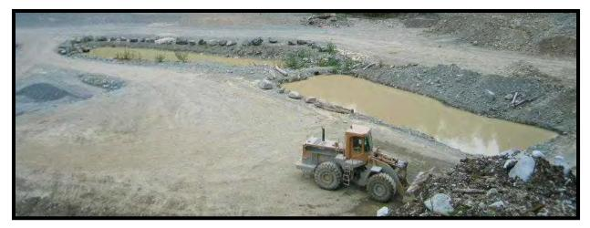
Figure 7-15: Settling Pond Example (Photo: City and Borough of Sitka)
