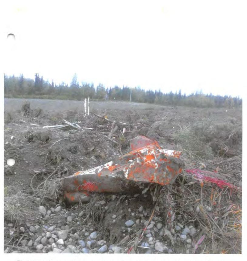
**CRUSHED SEPTIC TANK WITH CONTAMINATED SEWER ROCK DUMPED AND BURIED INTO SBC PIT SEPTEMBER 2014**
