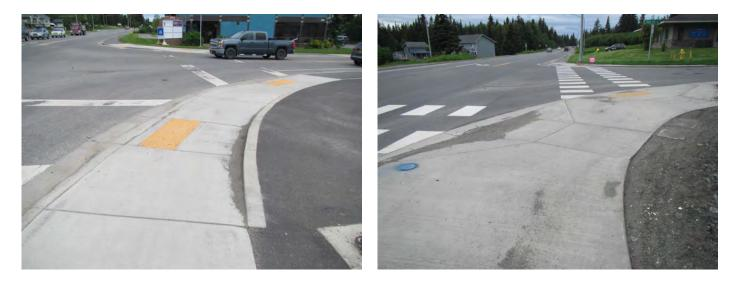
Figure 18: Curb Ramps that Direct the User into the Crosswalk
