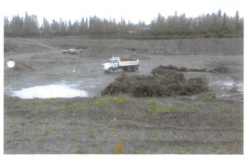
TRUCK DUMPING ORGANIC MATERIAL INTO THE OPEN WATER AQUIFER IN FLOOR OF SBC PIT SEPTEMBER 2014 21 January 2015
