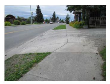
Figure 19: Driveway Entrance with Level Cross Slope
