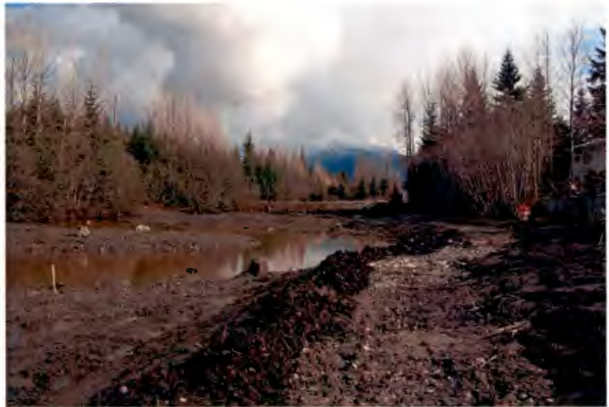
Glacier State shaped the rough trail bed and placed shot rock in May.
