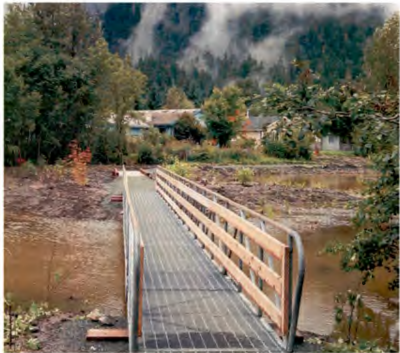
Right: The steel gangway donated by CBJ Ports and Harbors extends from the northwest end of the trail to the east side. Trail Mix built new cedar rails for safety.
