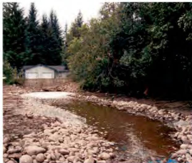
Glacier State returned to the outlet channel and dam 2 weeks after initial construction and added more cobble, lowered the dam elevation, and reshaped the channel.
