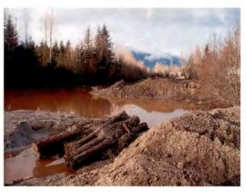
Early stages of filling in November, 2005. Logs are used to support machinery as the fill the fingers.
