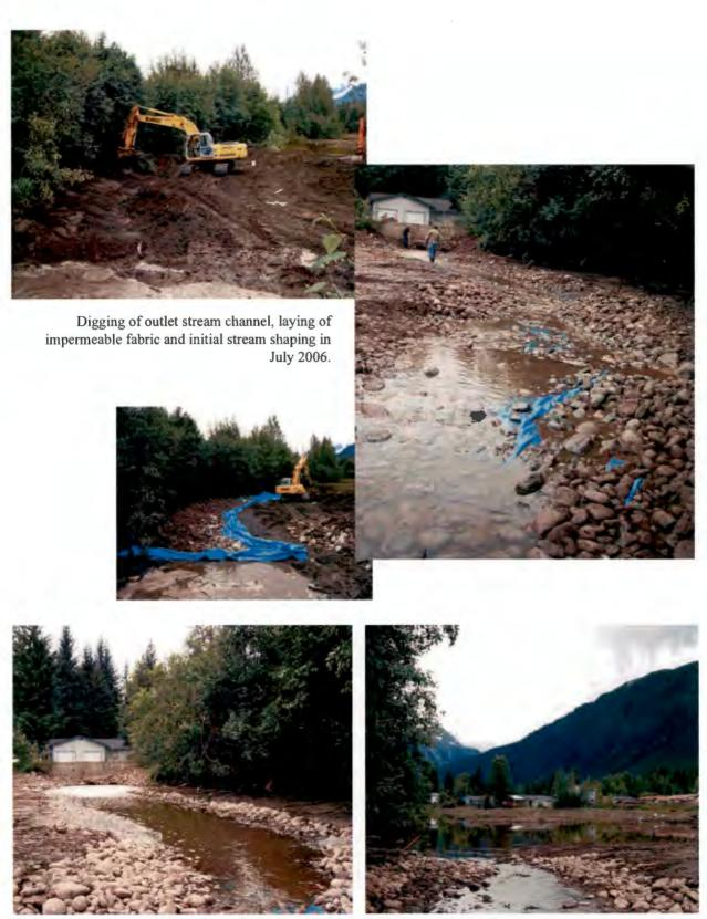
Glacier State returned to the outlet channel and dam 2 weeks after initial construction and added more cobble, lowered the dam elevation, and reshaped the channel.
