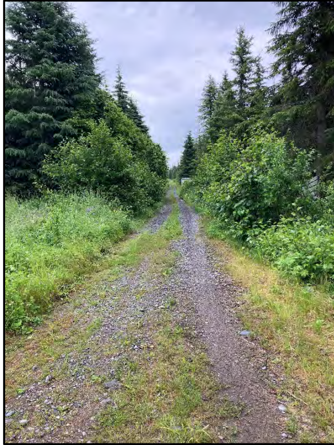
Figure A.4. Example of an unsurfaced road that has not been well maintained or frequently traveled.
