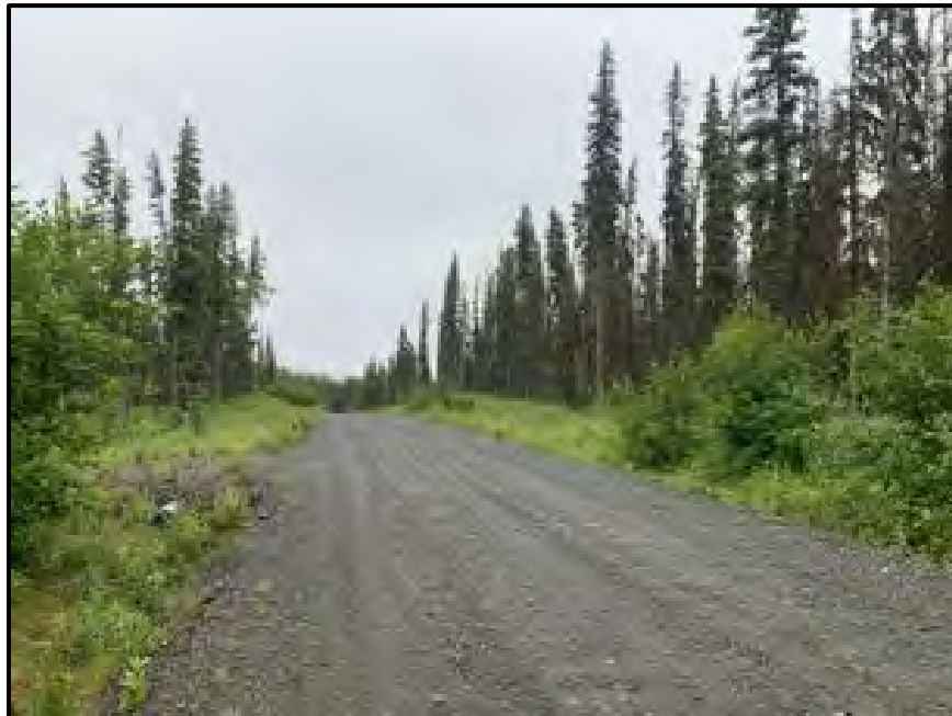
Figure D.28. Example of heavy vegetation along roadways.
