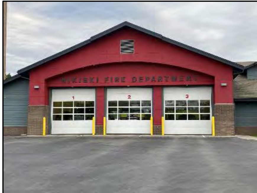
Figure D.23. The community is served by the Nikiski Fire Department.
