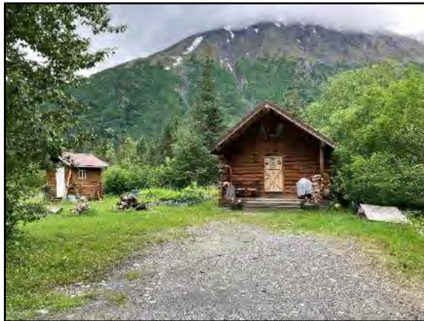
Figure D.7. Example of cabins and other values at risk with limited defensible space, suggesting fire response concerns.
