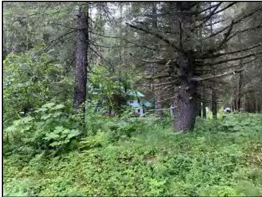
Figure D.3. Example of homes in Bear Creek with very minimal defensible space.
