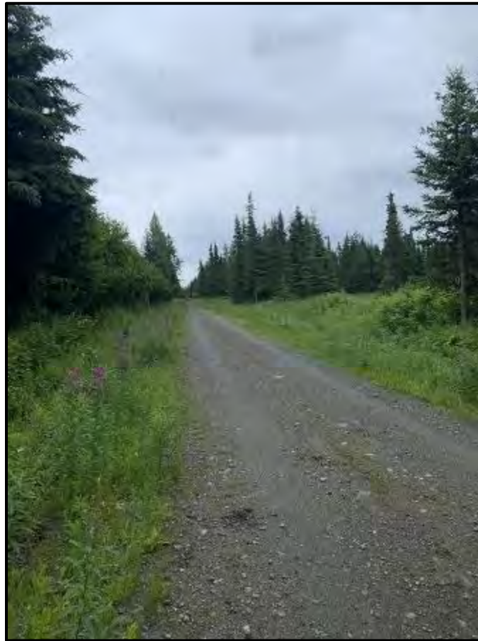
Figure D.4. Example of an unsurfaced road, a frequent occurrence within the community.
