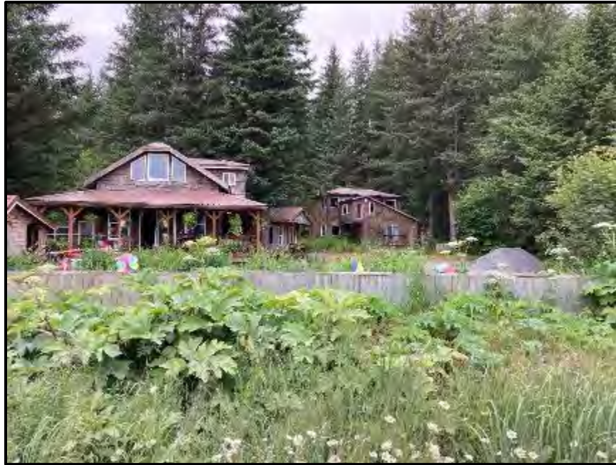
Figure D.20. Because the community is compact and encapsulated due to topography, many homes have limited defensible space or structure separation.
