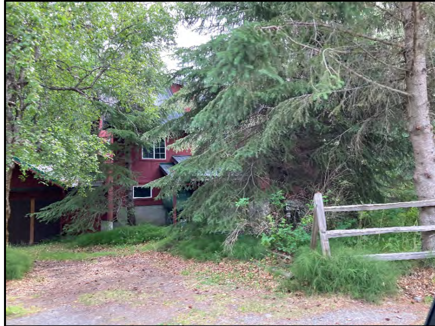
Figure 4.7. Example of poor defensible space.
