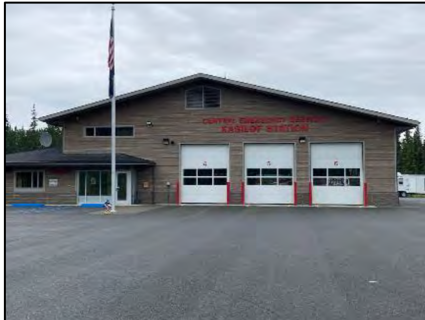
Figure D.18. The Central Emergency Services, Kasilof station serves the community.
