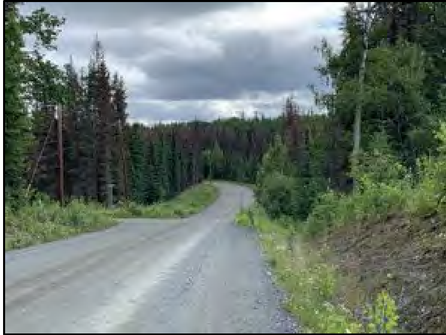
Figure D.32. Example of road conditions (narrow and unsurfaced) with limited defensible space.
